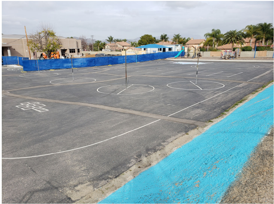
Photograph 1: North Hardcourt: Overall view of play area looking northeast.
