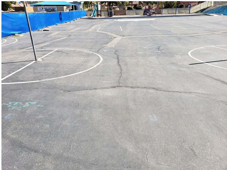
Photograph 2: North Hardcourt: View of play area looking east. Open cracks and previously patched cracks.
